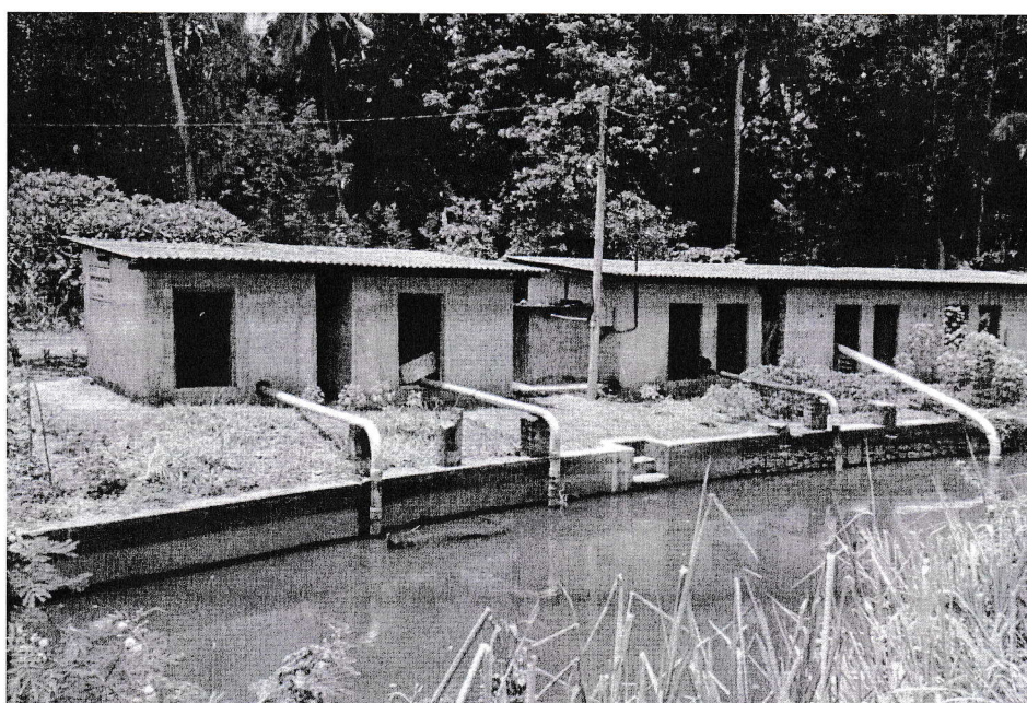
Figure 2: Pump houses near the main water channel
