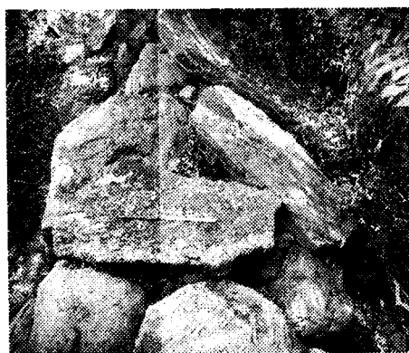
Photo 3. This is the Neeli Bemma primitive dam of Kala Oya which has been built by using shapeless rough rock blocks and slabs
