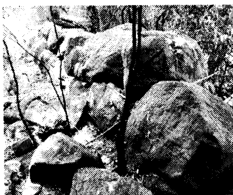
Photo 3. This is the Neeli Bemma primitive dam of Kala Oya which has been built by using shapeless rough rock blocks and slabs
