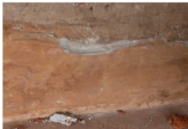
Figure 5. Outer plaster of the square chamber of Jethawana sthupa.
