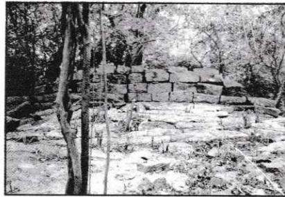
Yakabemma dam at Yan Oya
