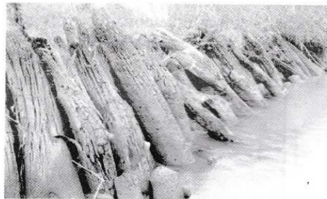
Timber made dams at Deduru oya
